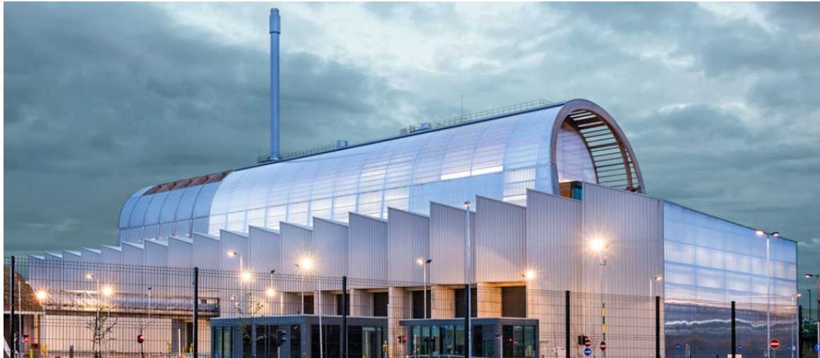
Figura 15 – Leeds Recycling & Recovery Centre ( www.danpal.com )
